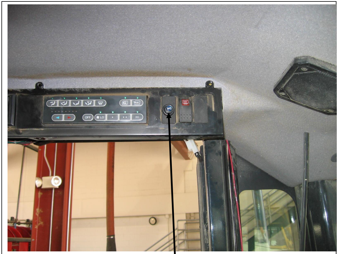
A/C on off switch mounted beside heater control panel.
